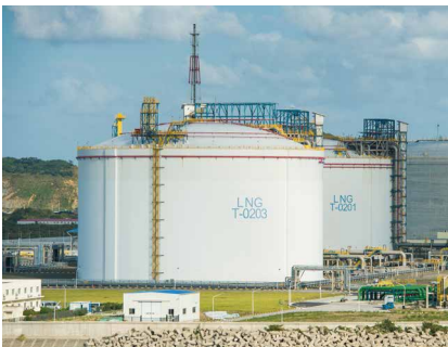
Liquid level tank
